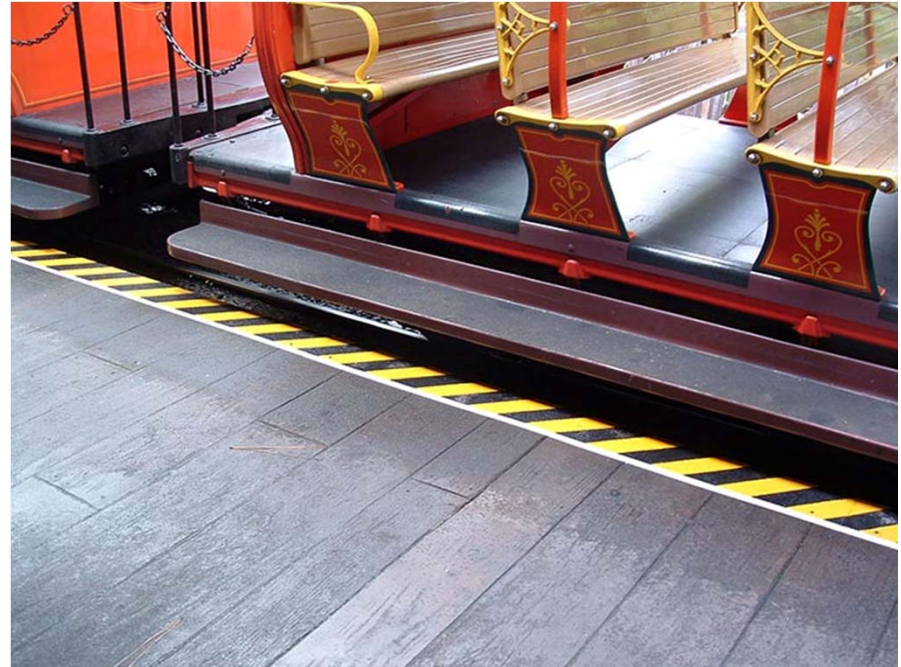
BOLD STEP® Hazard Plates Installation
